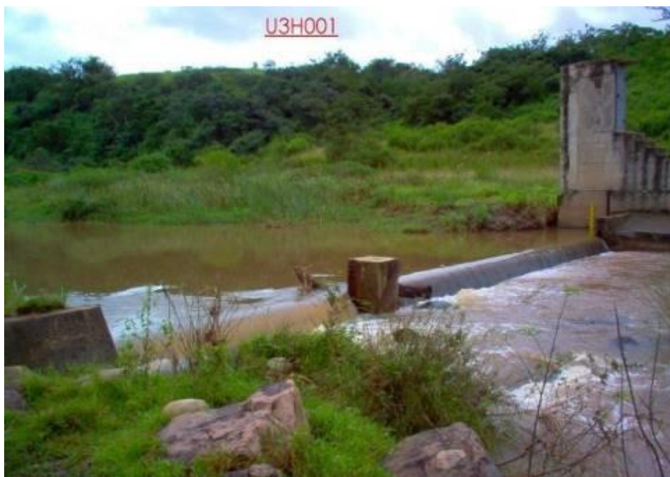
Figure 3.2 Example of a flow gauging weir on the Tongati River at Riet Kuil (DWS 2015)
